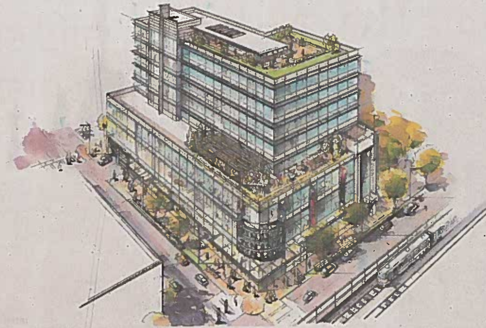
A rendering of the nine-story, mixed-use building that is planned for 38-01 Queens Blvd. in Queens.
